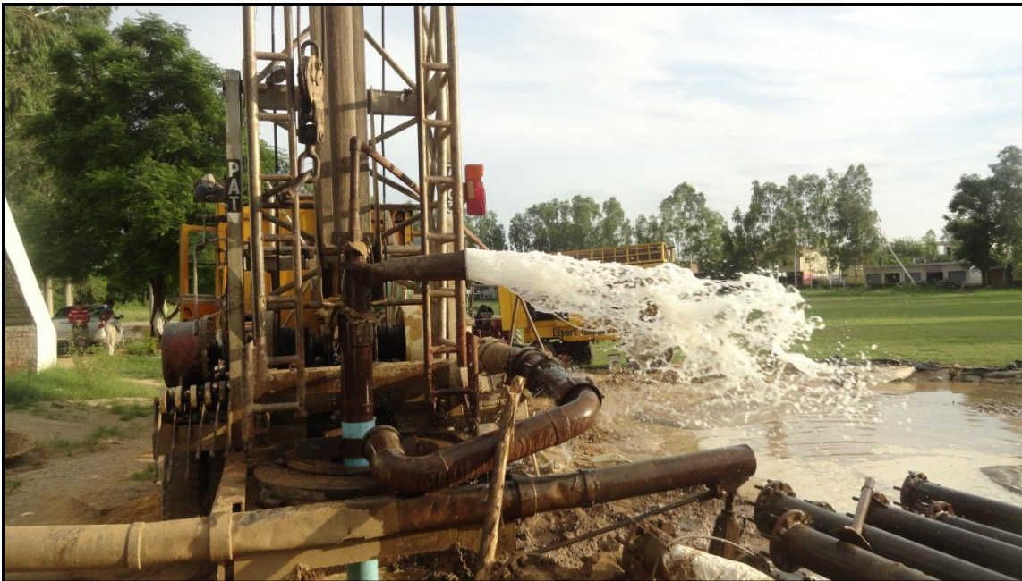
Photo 4.3d: Installation of piezometer on the selected site
