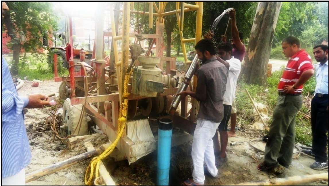
Photo 4.3b: Installation of piezometer on the selected site
