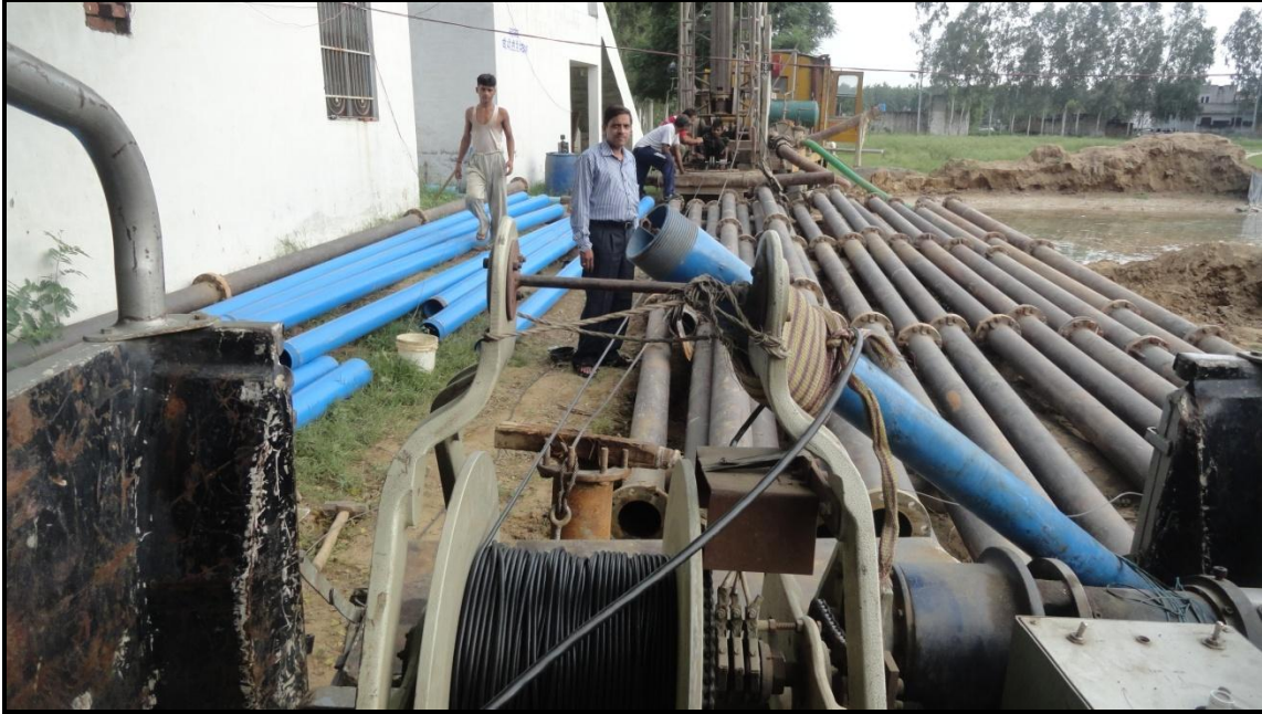
Photo 4.3c: Installation of piezometer on the selected site
