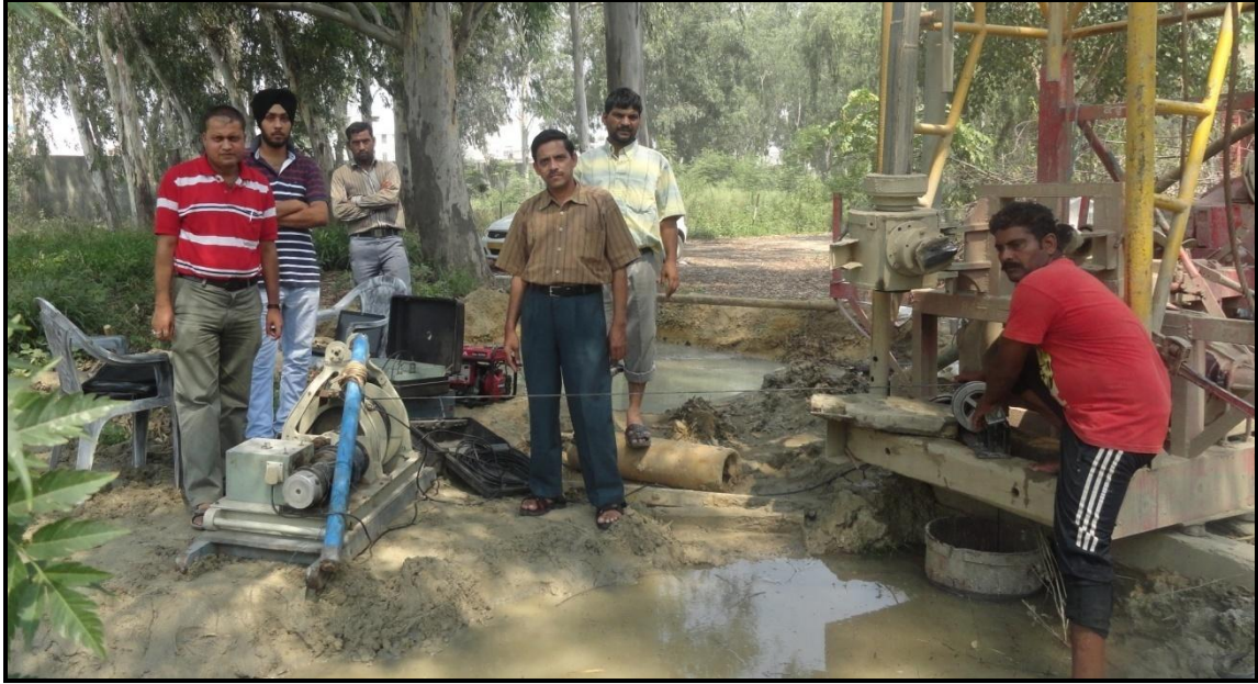
Photo 4.3a: Installation of piezometer on the selected site
